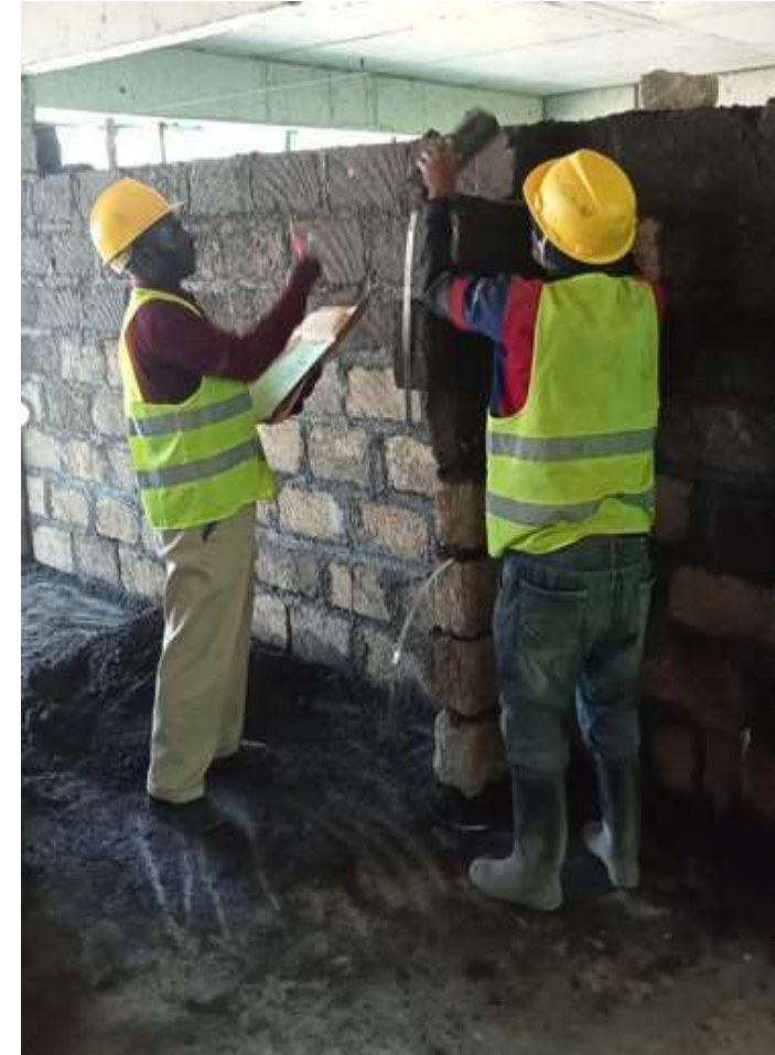
Masonry Onsite RPL Assessment
