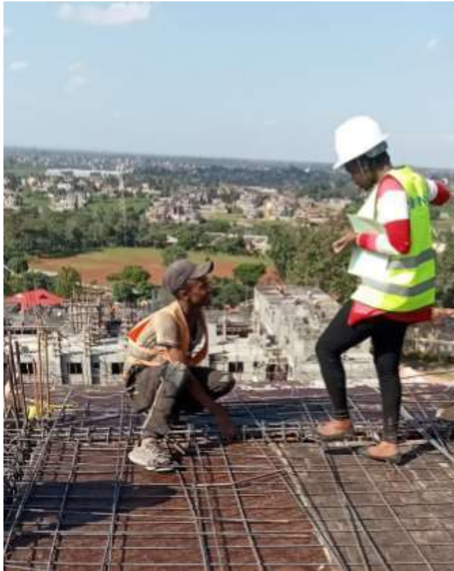
Steel Fixing Onsite RPL Assessment
