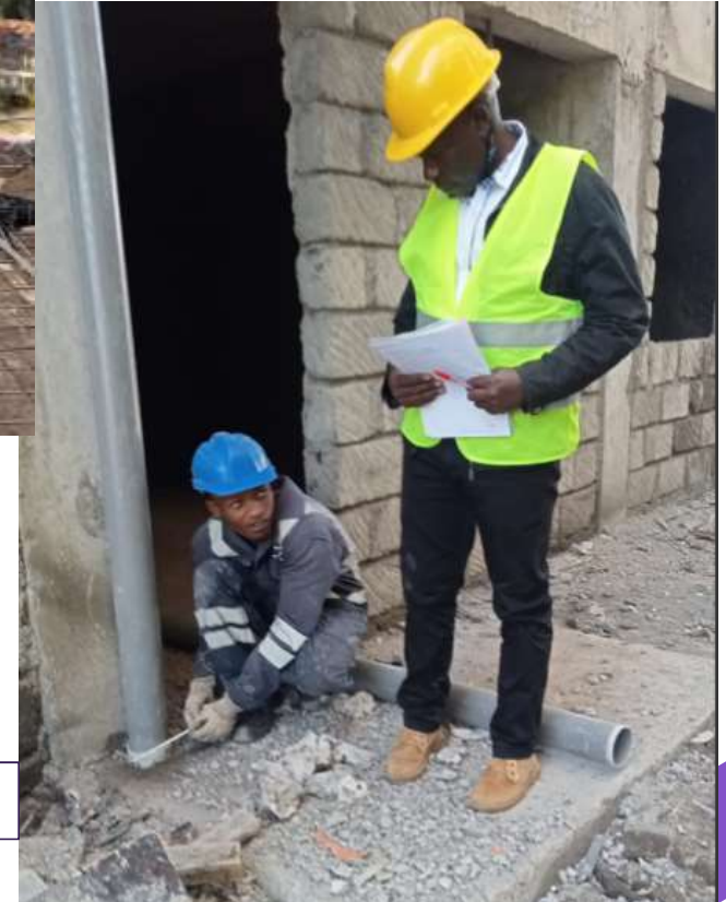
Plumbing Onsite RPL Assessment
